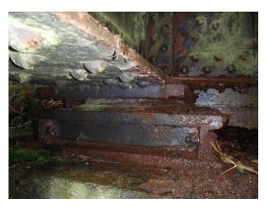
Surface Corrosion on Bearings
