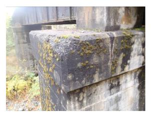
Spall on NE corner of Pier 2
