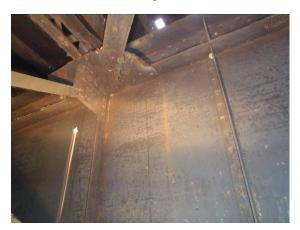
Corroded Gusset Plate inside Girder
