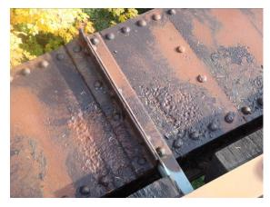
Top Plate of Top Chord Pitting (Deck Truss Span)
