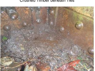
Debris on Bottom Flange Angles (Typical)
