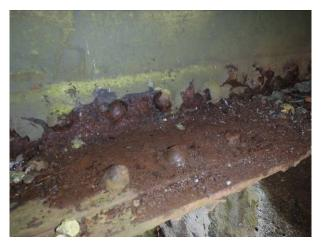
Corrosion of Bottom Flange Angle (Typical)
