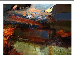
Corrosion on Bearing (Typical)
