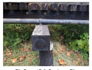
Pile Cap not Fully Bearing on Pile
