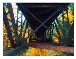
Corrosion on Secondary Bracing Members
