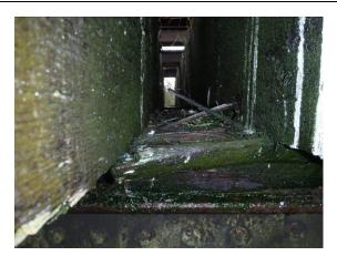
Crushed Timber beneath Ties
