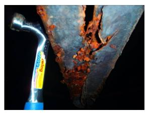
**Corroded Lateral Bracing Members**
