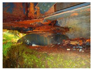
Corroded South Bearing (Typical)
