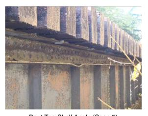
Bent Top Shelf Angle (Span 5)
