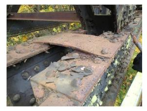
Bowed Plate on Bottom Chord of Truss
