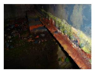
Corrosion on Bottom Flange of Bottom Chord
