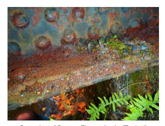
Corrosion of Bottom Flange Angle (Typical)
