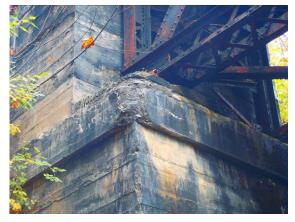
North Abutment Spalling
