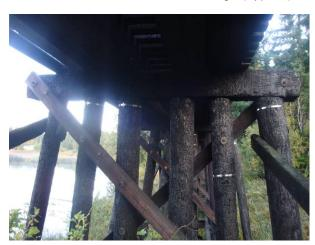
Fire Damage of Pier (Typical)
