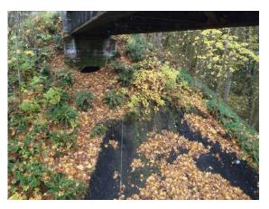
Slope Erosion in front of South Abutment
