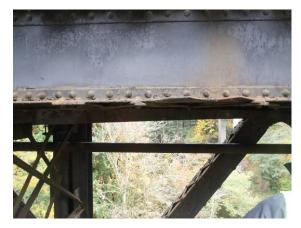
Bent Truss Flange from Installation Jacking
