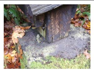
Split Base of Intermediate Timber Bent
